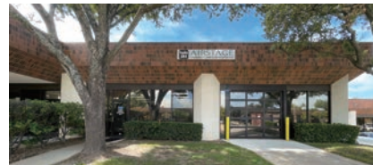
North America R&D Center (USA)
