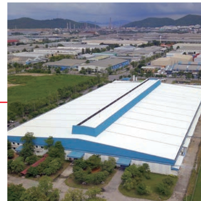
Fujitsu General (Thailand) Co., Ltd. (Thailand) Factory-2
