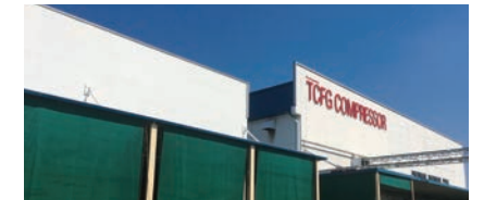
TCFG Compressor (Thailand) Co., Ltd. (Thailand)
