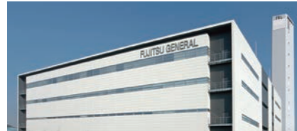
JAPAN Head office, R&D center and 60 m height difference testing tower (Japan)
