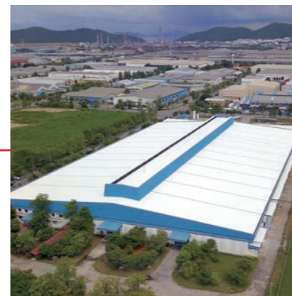
Fujitsu General (Thailand) Co., Ltd. (Thailand) Factory-2
