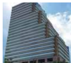
Fujitsu General (Thailand) Co., Ltd. Bangkok Office (Thailand)
