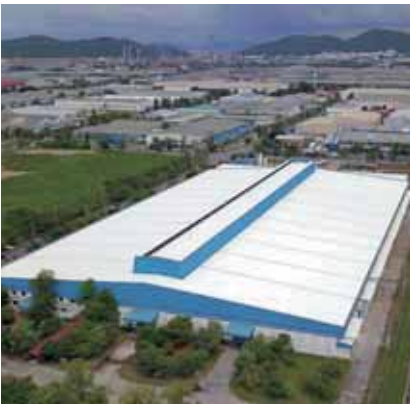
Fujitsu General Co., Ltd. (Thailandia) FACTORY-2
