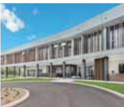
Fujitsu General (Aust.) Pty Ltd. (Australia)
