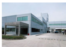
FUJITSU GENERAL (SHANGHAI) CO., LTD. Technical Center
