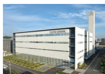
Kawasaki Headquarters/ Air Conditioner Technology Building
