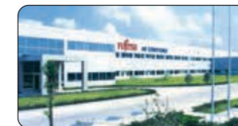
Fujitsu General (Shanghai) Co. Ltd.
