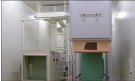
Air Volume Measurement Room
