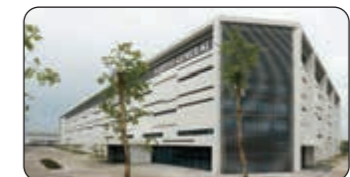
New Engineering and R&D Centre in Thailand
