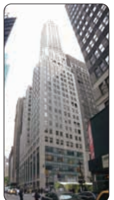
Fujitsu General Solution Centre "THE AIRSTAGE"
