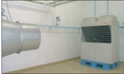
Shower Test Room
