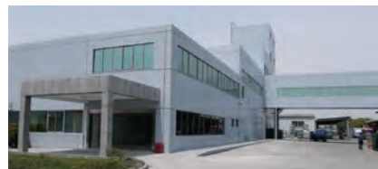
R&D center in Fujitsu General (Shanghai)
