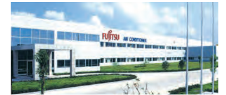
Fujitsu General (Shanghai) Co., Ltd. (China)
