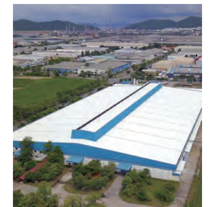
Fujitsu General (Thailand) Co., Ltd. (Thailand) Factory-2
