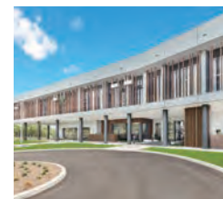
Fujitsu General (Aust.) Pty Ltd. (Australia)
