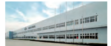
Fujitsu General Central Air-conditioner (Wuxi) Co., Ltd. (China)
