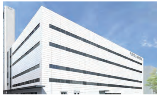
Technology research building (Japan)
