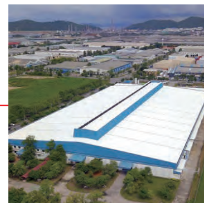
Fujitsu General (Thailand) Co., Ltd. (Thailand) Factory-2
