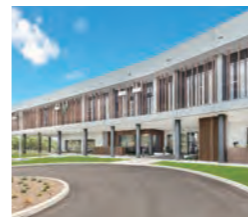
Fujitsu General (Aust.) Pty Ltd. (Australia)
