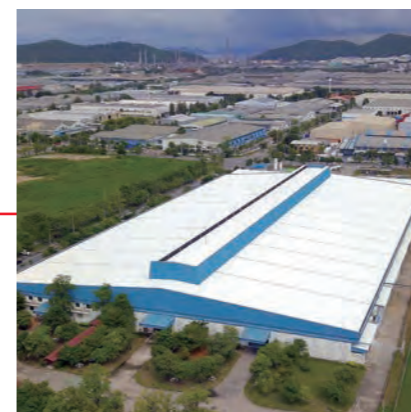
Fujitsu General (Thailand) Co., Ltd. (Thailand) Factory-2
